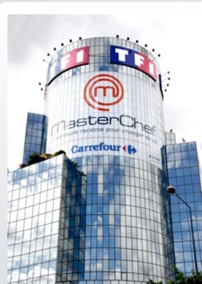
DECALS ON TFI BUILDING
