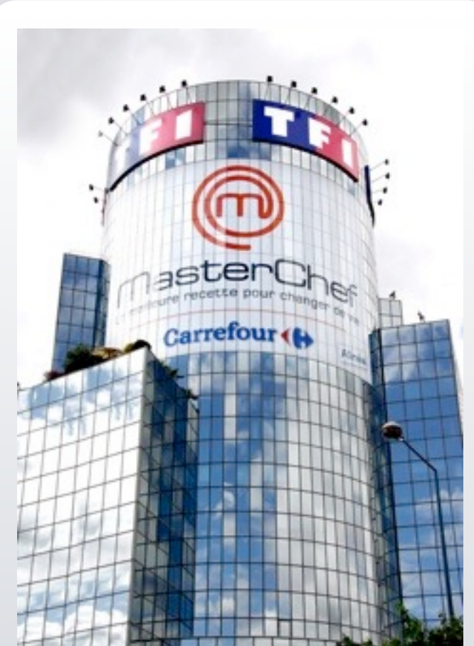
DECALS ON TFI BUILDING
